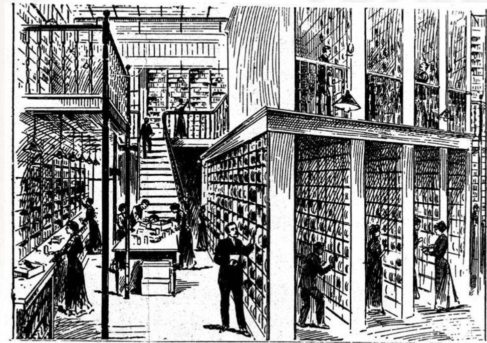
COLUMBIA COMPANY'S RECORD STORE WITH A CAPACITY OF 300,000 RECORDS.
