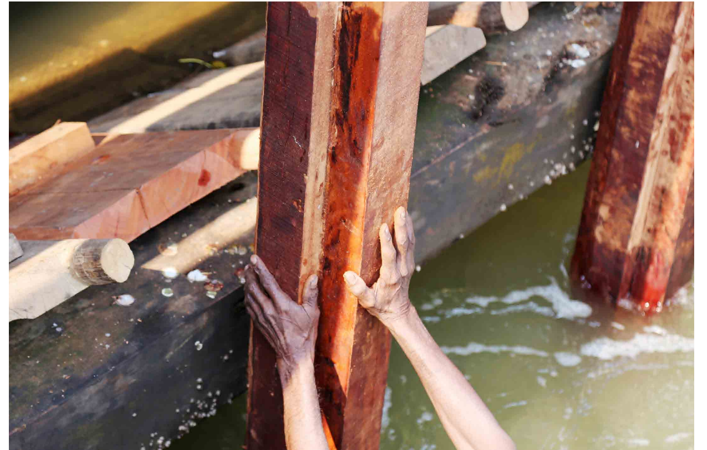
Fisherfolk and people from the village gather during low tide to give a hand when it is time to replace the old doors eaten by wood borers, mud crabs and clams; Britona (2023) | From the Foundation Project with Amrita Barua
