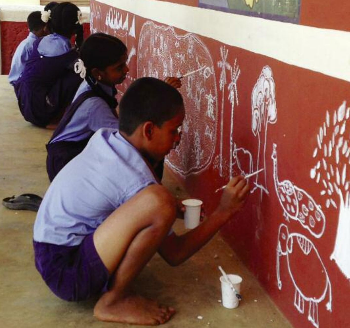
Students painting the wall of the Cluster Resource Centre, Tallur Cluster, Baindur Block, Udupi district as part of a grant made to Ganapathi Hoblidar.
